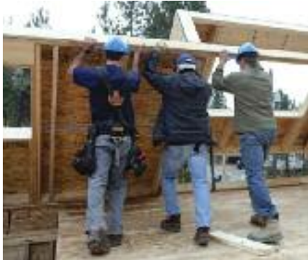
Volunteers raising a wall at Elk Road building.
